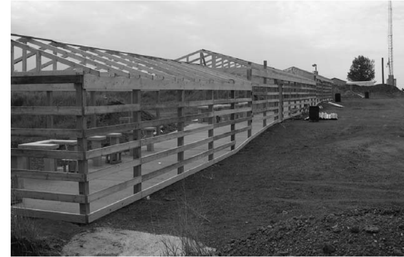
Constructions is going fast. Don't delay getting your access card.
